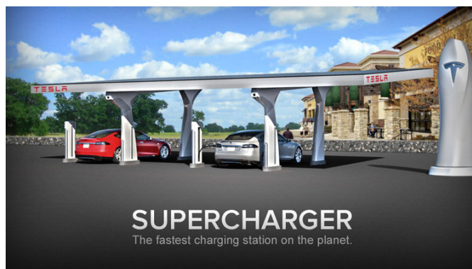
Fig. 2 TESLA supercharge EV charging station (Image: TESLA).
