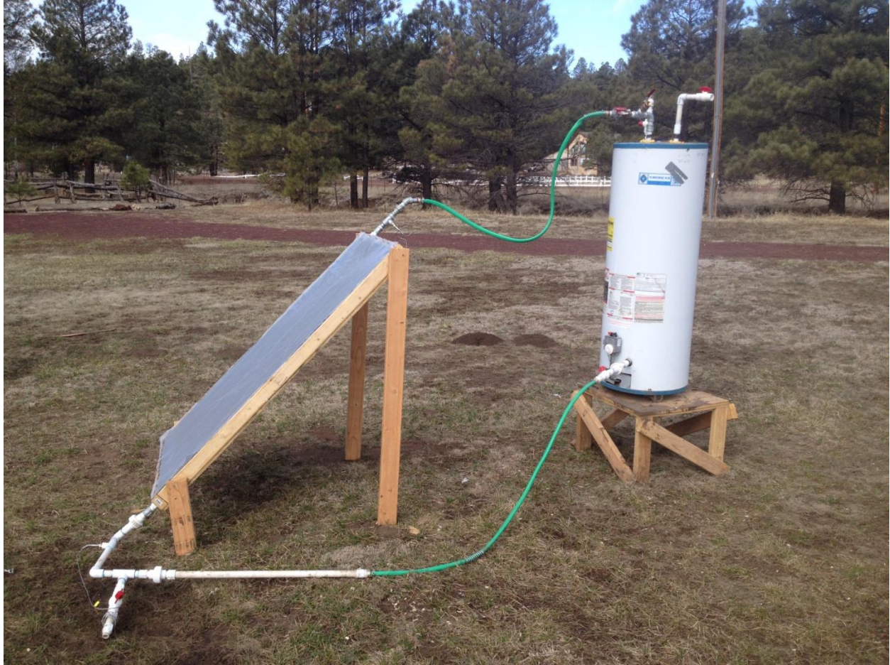
Figure 8: Tank to collector integration
