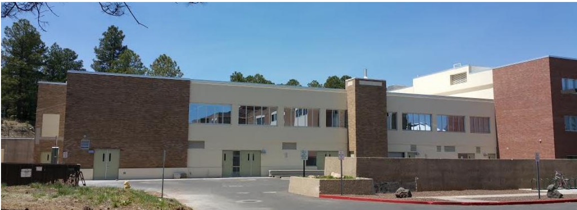
Figure 1: East Wall of the NAU Engineering Building
