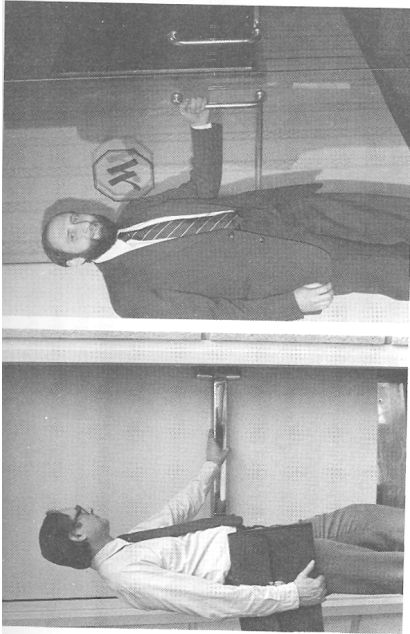
1.5 Affordances of Doors. Door hardware can signal whether to push or pull without signs. The flat horizontal bar of A (above left) affords no operations except pushing; it is excellent hardware for a door that must be pushed to be opened. The door in B (above right) has a different kind of bar on each side, one relatively small and vertical to signify a pull, the other relatively large and horizontal to signify a push. Both bars support the affordance of grasping: size and position specify whether the grasp is used to push or pull—though ambiguously.
